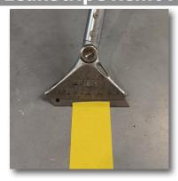
Begin LeanStripe removal with a scraper. Getting under the LeanStripe with the scraper, peel up 1-2 inches (2-5 cm) of striping.
