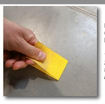
Peel off tape at a **steep** angle (not at 90°) to minimize residue left on the floor.
